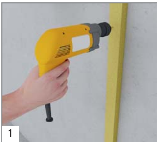
1 Pre-drill the holes for the mechanical fixings (diameter: 6 mm).
