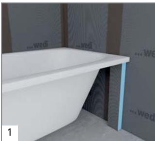
1 Fit the support in the wall area.
