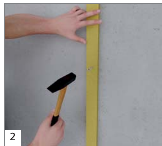
2 For connection to the wall, vertically attach the wall and door fixingset by using mechanical fixings.
